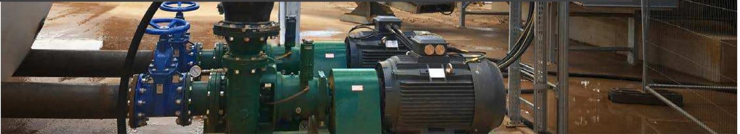
Pioneer standard centrifugal pumps provide superior performance in a variety of high pressure, sewage, trash or dewatering applications. The large stainless-steel impeller eye yields lower NPSHr and improved vapor-handling capabilities, making them ideal for industrial, municipal, agricultural, mining, and oil and gas settings.
